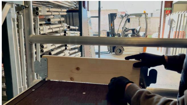
3. Place the first long board at an angle to facilitate anchoring, as shown in photo 2.
